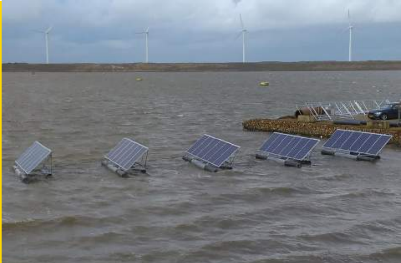
January 2016: Start of Slufter solar panel test project
