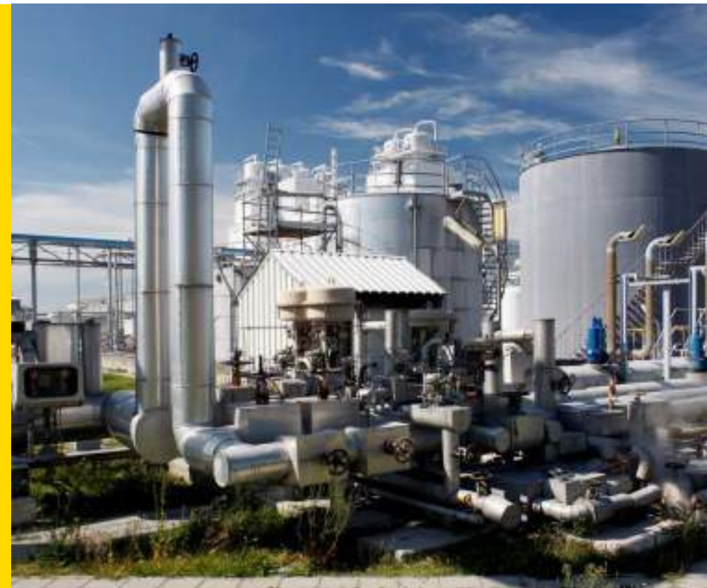
Botlek Steam Pipe
